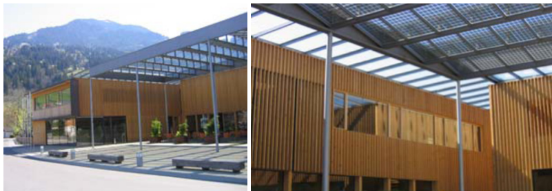
Integration of solar cells into a building construction: Gemeindezentrum, Ludesch, Austria (photo Ulla Jansson)
